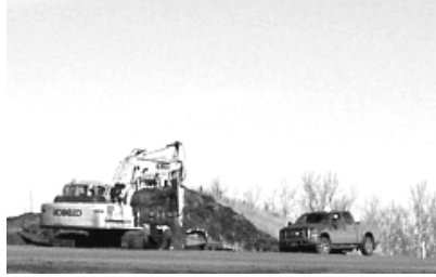
Crews working on the new water supply line north of Bashaw.
